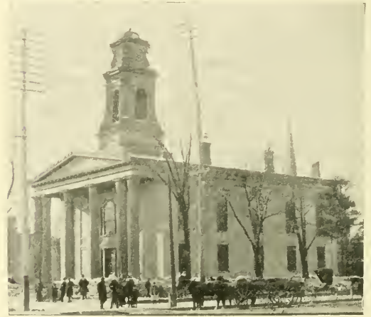
OLD COURT HOUSE.
